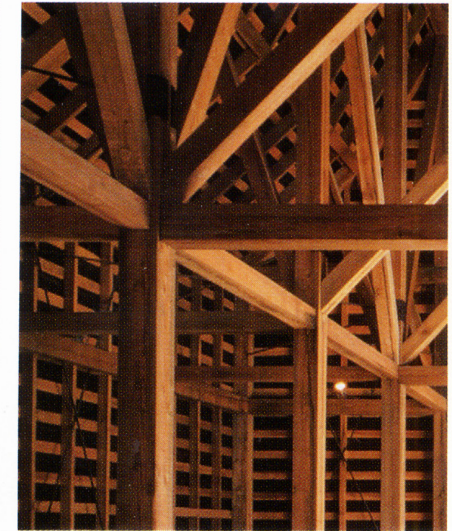
Photo 7. The area for the wood and metal shop with the central 8x8 columns and 8x8 cross beams extending to the right. Cross beams between columns and those extending left to the north wall are 4x4s.
