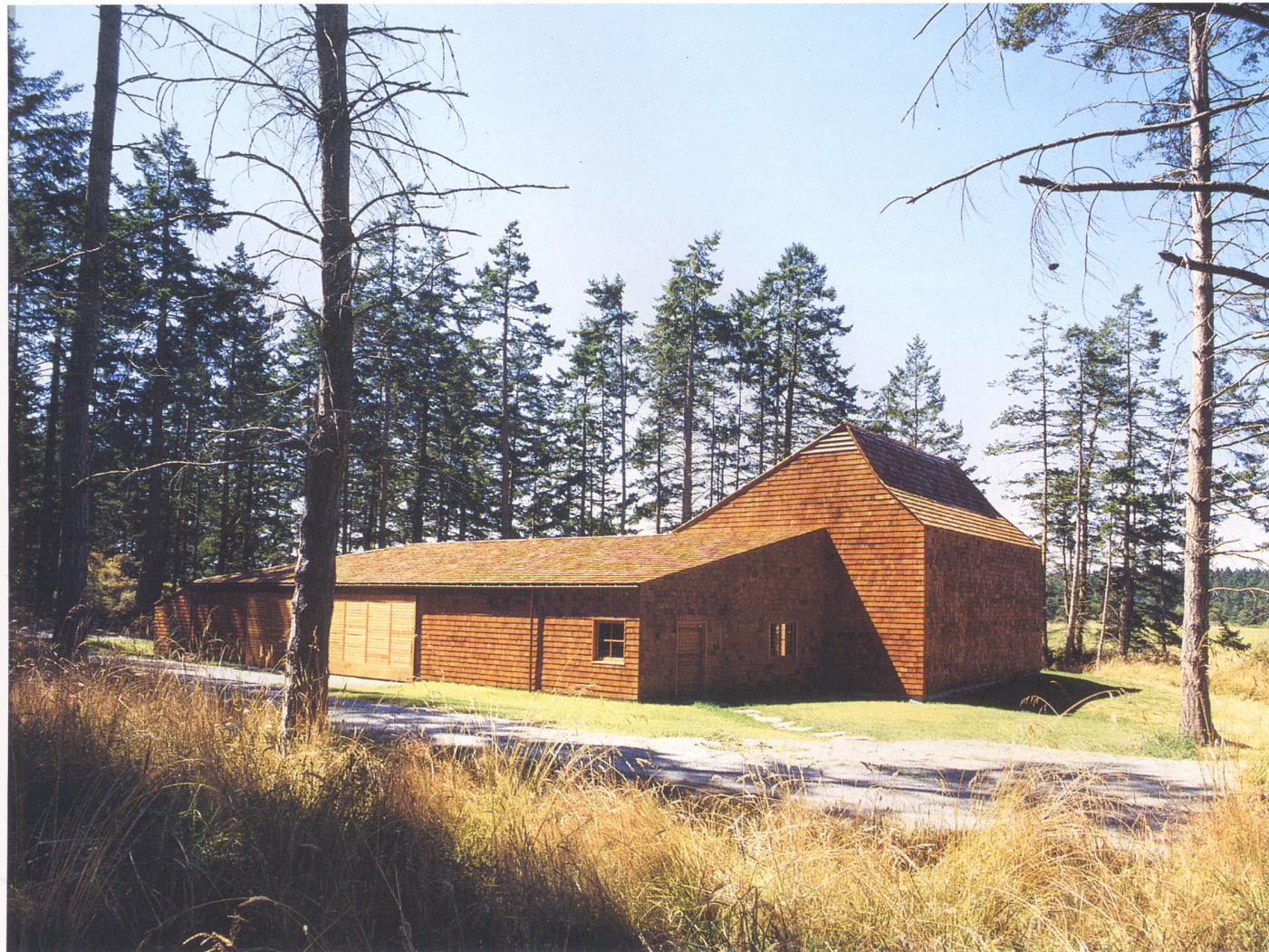
Photo 5. View from the east showing western red cedar roof shakes and wall shingles, and roof angles.
