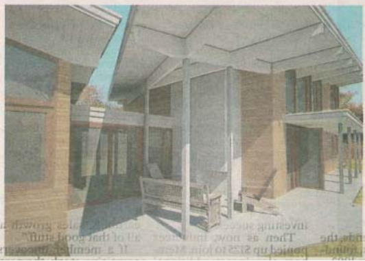
FINE FIT: The HingeHouse is 'like a big Lego building system,' so it can be adapted for an individual site or buyer, says Cambridge architect Maryann Thompson, above. Her designs range from the two-bedroom home on beachfront property she showcases above to the larger home seen at left. She says 10 homes are now in development.
